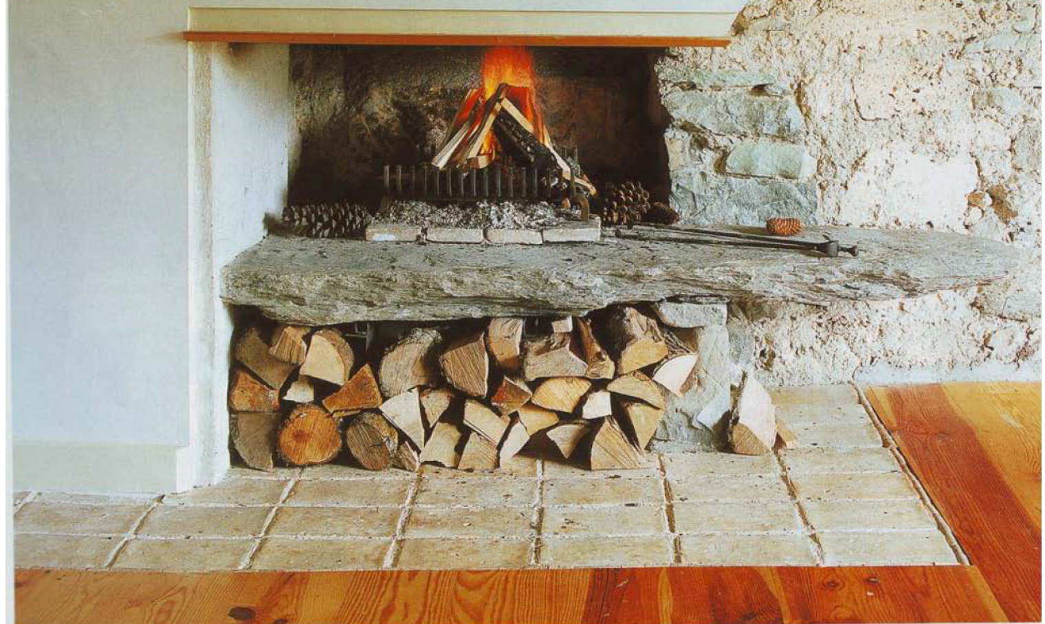
The fireplace was inspired by Alvar Aalto's Villa Mairea in Finland and is made from plasterboard. The stone
