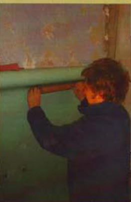
From left, a ghostly figure behind the polycarbonate sheeting; Rob uses a rolling pin to smooth linoleum over a drainage pipe in the bathroom; Rob in the new fireplace mid-construction; John outside the house during their first winter there before work had begun on the front elevation
